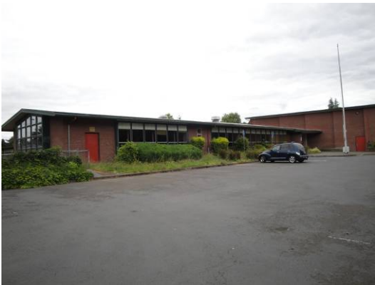
West elevation entry
