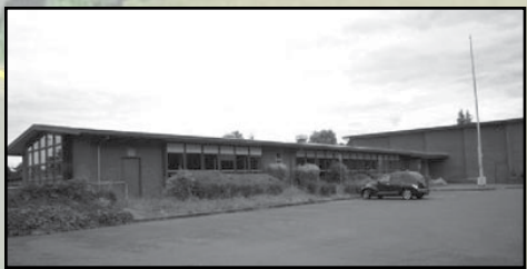
2009 photo of West elevation
